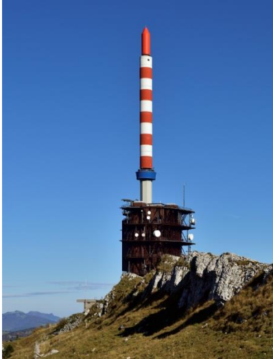
Mobilfunkantenne (Chasseral) © Keystone/M. Jegerlehner
